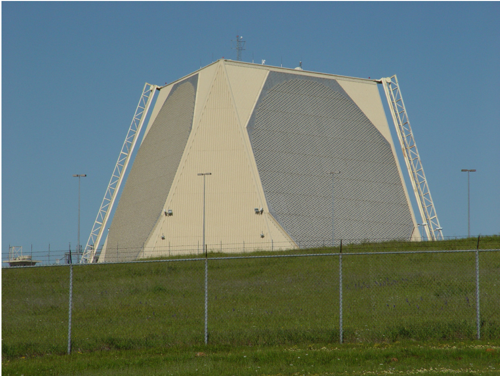
Figure 9: The PAVE Phased Array Warning System (PAVE PAWS) at Beale AFB employs a pair of Raytheon AN/FPS-115 phased antenna arrays comprising several thousand smaller antenna elements. Its electronically steered beam is capable of detecting submarine launched ballistic missiles at ranges up to 3500 nmi (6500 km) with 2.2° azimuthal precision . Source: Missile Defense Agency
